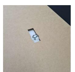
Close up of installed screw and eye Screw in the plaster mate plug until its in fully
