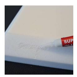
Step -1 apply the supa glue Apply supa glue to the beveled edge about 50mm down from the top corner on both sides
